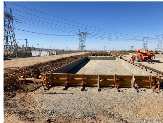
Forms Built and Ready for Rebar Installation
