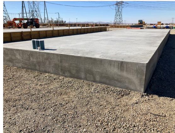
Close Up Poured Foundation
