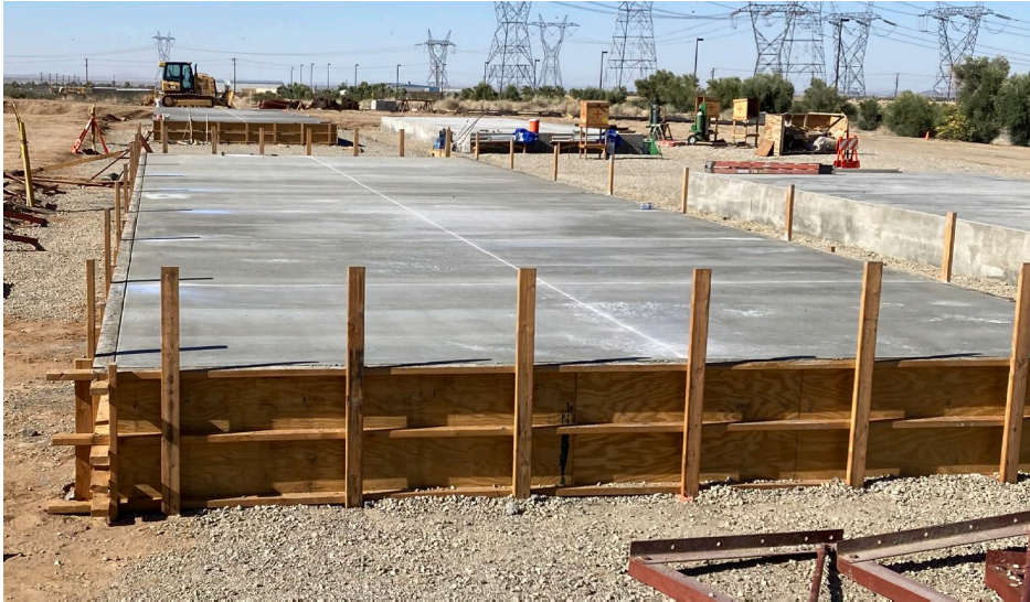
5 of 12 Foundations Poured
